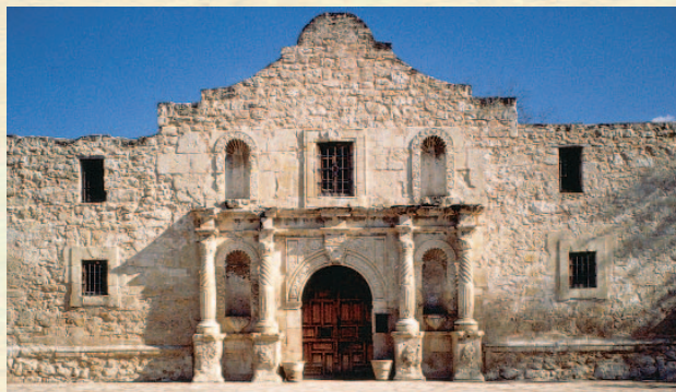
The restored Alamo today
